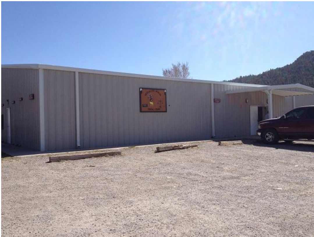
➤ Mescalero Apache Tribal Court Building
